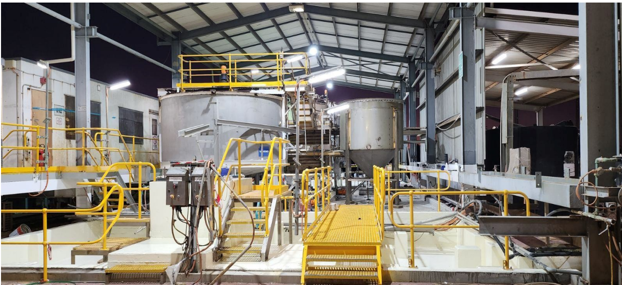
Figure 2: Refurbished SX plant at Cloncurry Hub
