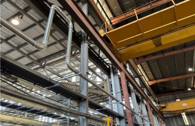
Figure: LPG gas piping installed
