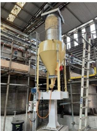
Figure: Hydromet piping progressing (left) Vortex pre-mixer installed and terminated (right)
