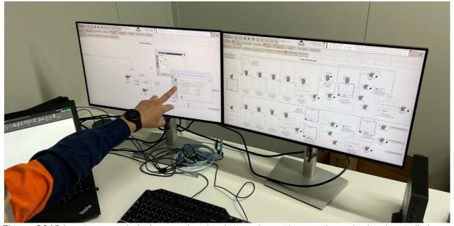
Figure: SCADA system commissioning ensuring signals to equipment is correctly received and controlled.
