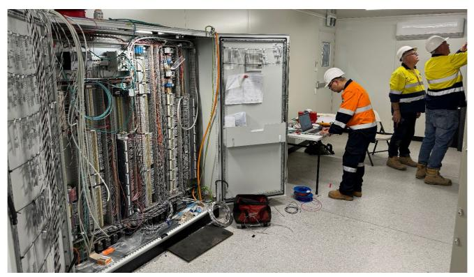
Figure: Commissioning process control systems with Rockwell representative on site.
