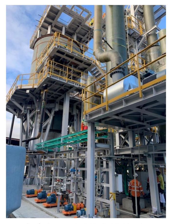
Figure: Spray Roaster area nearing mechanical and electrical installation complete
