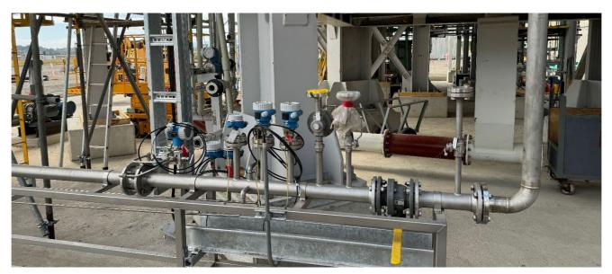
Figure: Instrumentation installed for Spray Roaster
