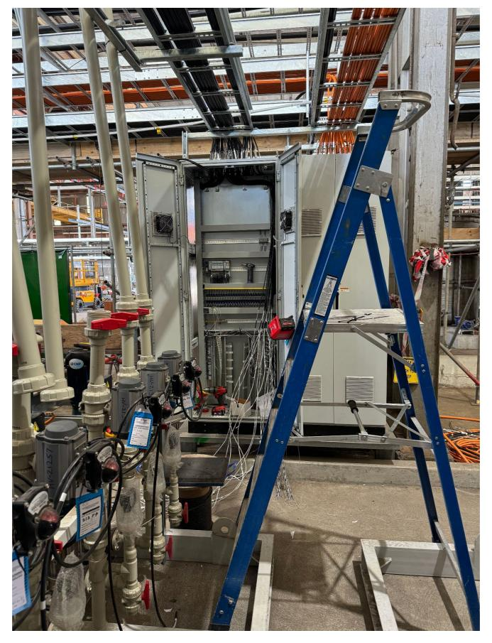
Figure: Terminations completed for the control cabinets in the Filtration area
