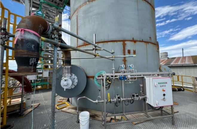
Figure: Spray Roaster piping and burner system installed
