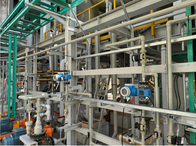
Figure: Spray Roaster instrumentation installed, ready for termination
