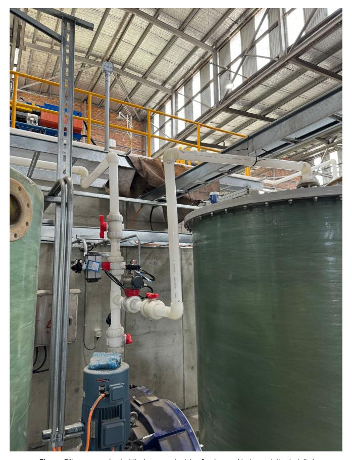
Figure: Filter area mechanical (tanks, pumps), piping & valves and instrumentation installed
