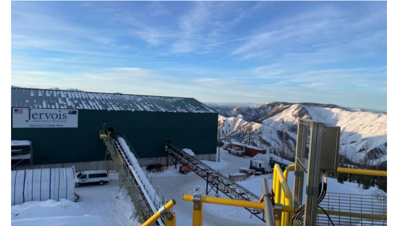
Surface construction (January 2023)
