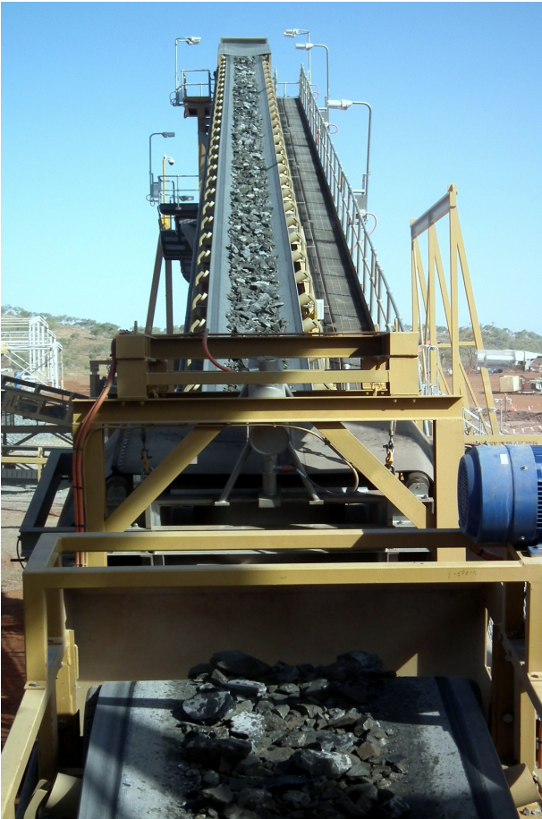
Figure 2: Conveying ore from the Primary Jaw Crusher to the screen above No 1 Rolls Crusher
