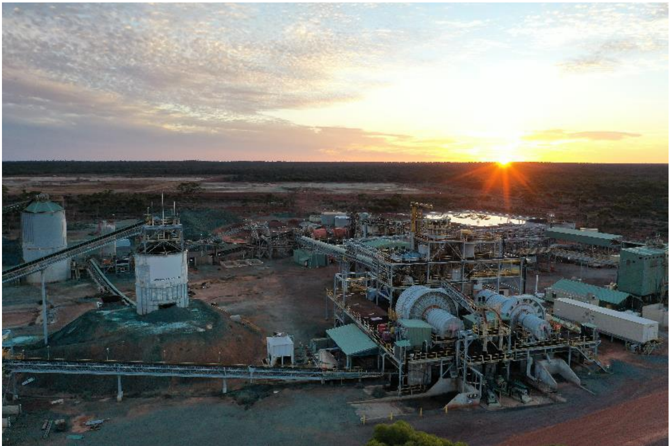
FIGURE 1 – BLACK SWAN 2MTPA PROCESSING PLANT
