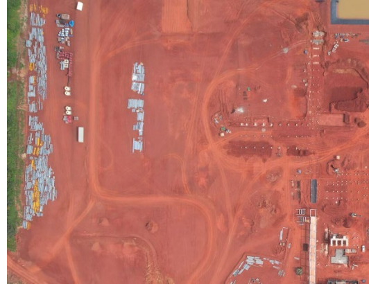
Image 9 - Materials and wet plant footings
