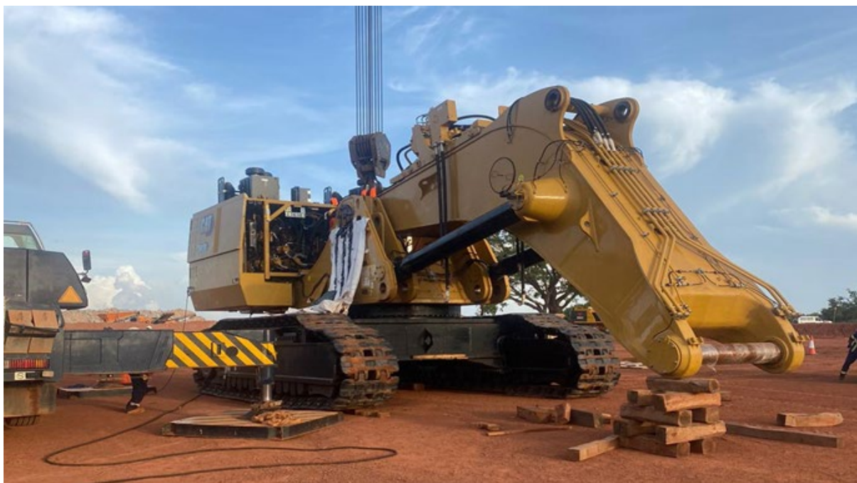
Image 2 - Construction of Cat 6030 Excavator which arrived on site
