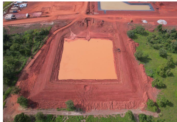
Image 7 - Plant drainage and sediment pond
