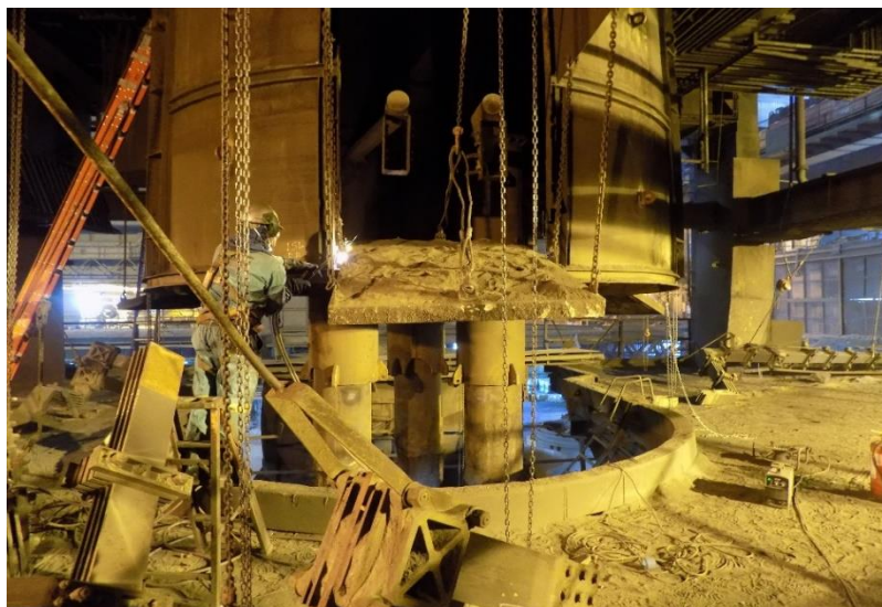
Figure 3 and 4: Dismantling of equipment at Transalloy's site
