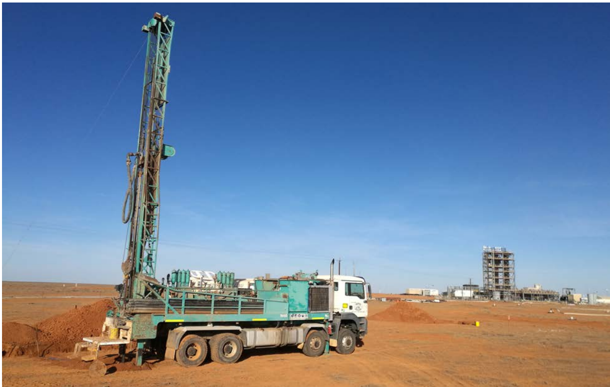
Figure 2: Photograph showing drilling operations in close proximity to the processing plant.
