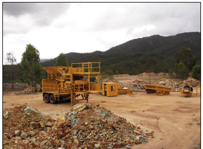
Picture 15: Primary crusher ready for final assembly.
