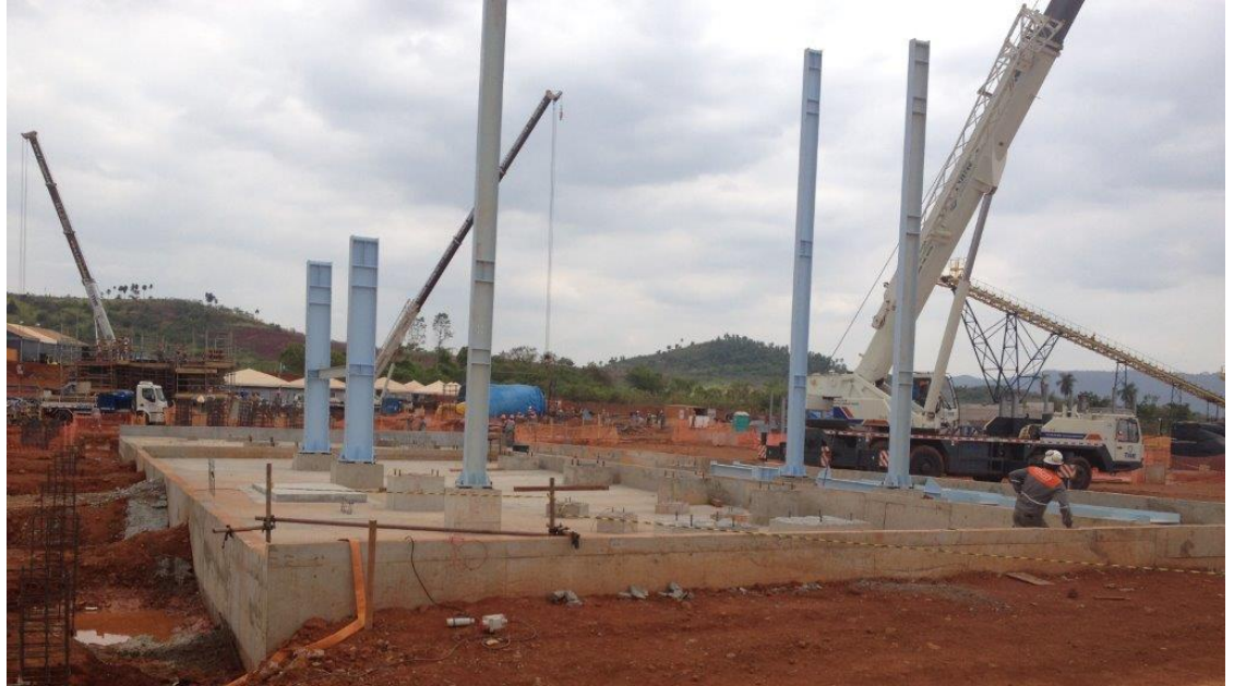
Flotation floor civils are sufficiently advanced to allow the start of structural steel which will support the float cells
