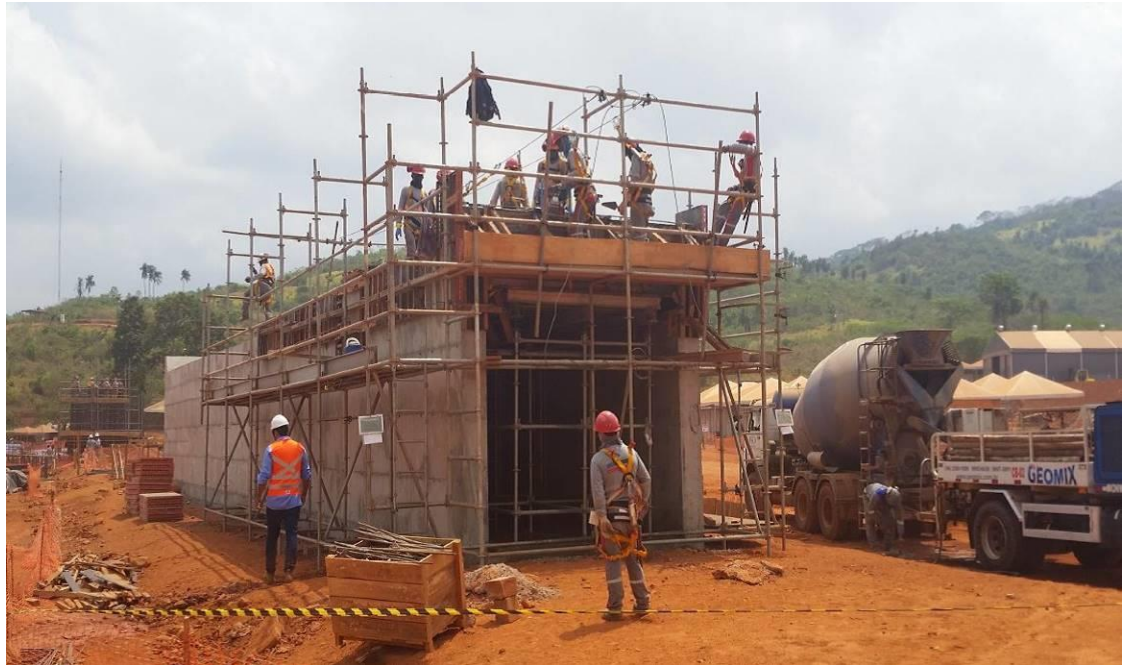
The Ball Mill feed reclaim tunnel civils are completed
