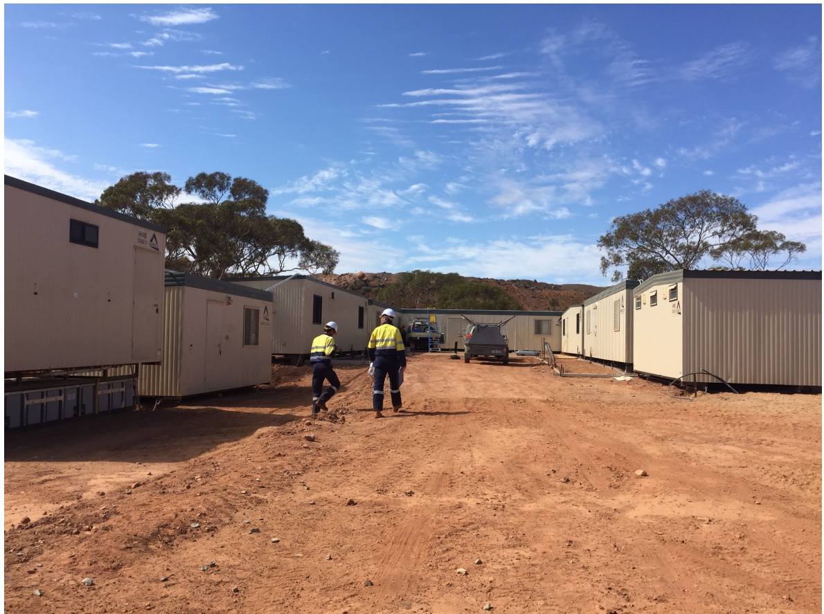
Figure 2: Site office set-up in progress.
