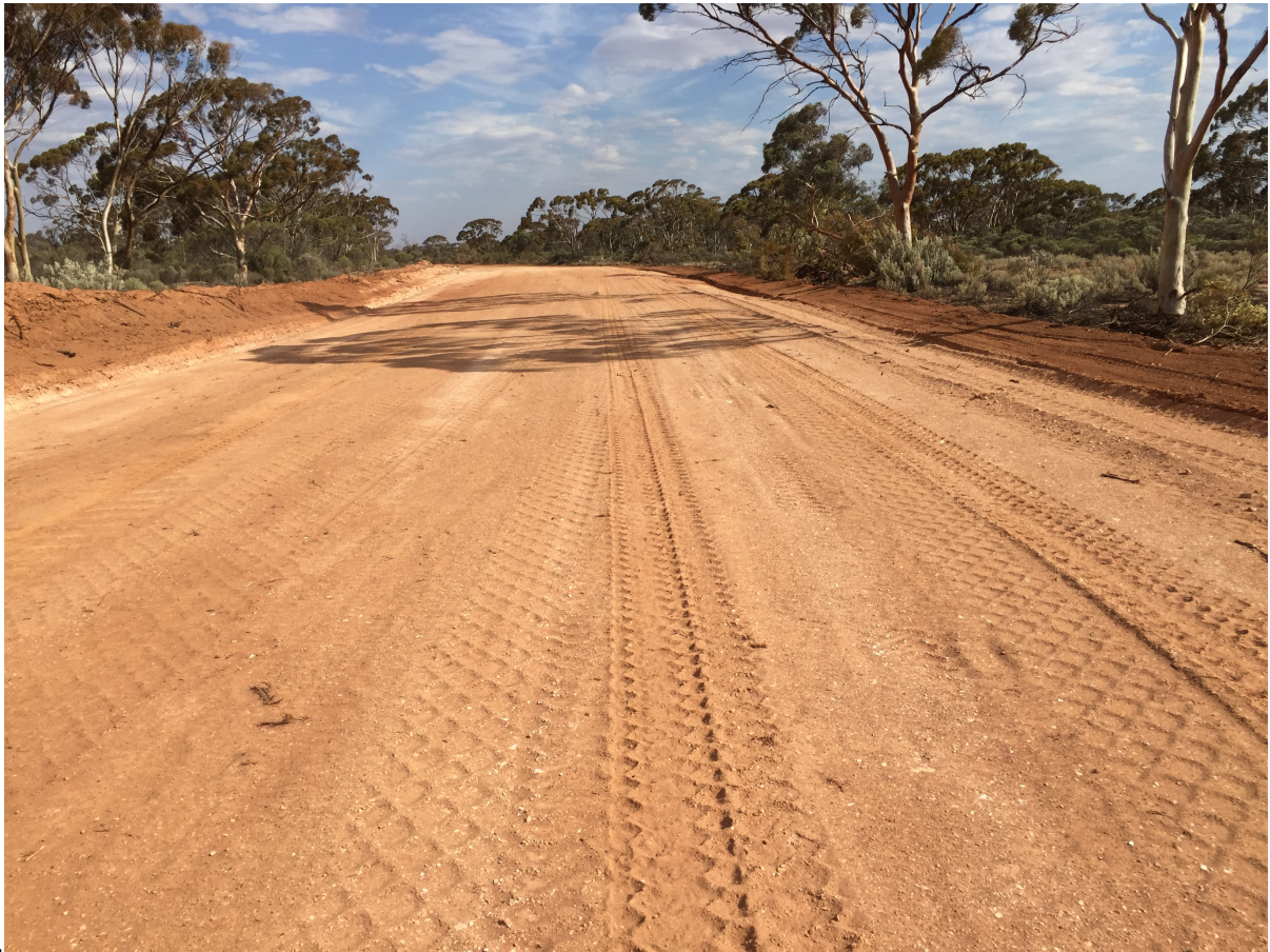
Figure 3: Haul road clearing completed in preparation for road construction.
