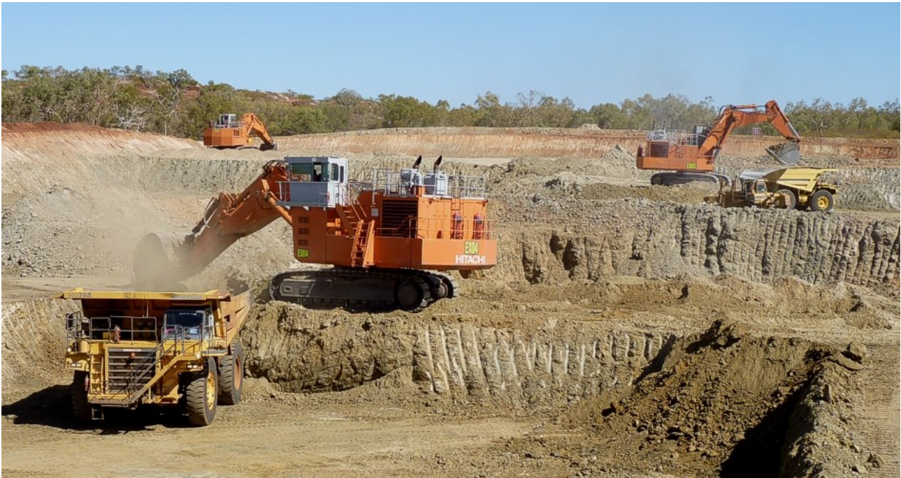
Figure 2: Mining commences at Las Minerale Starter Pit
