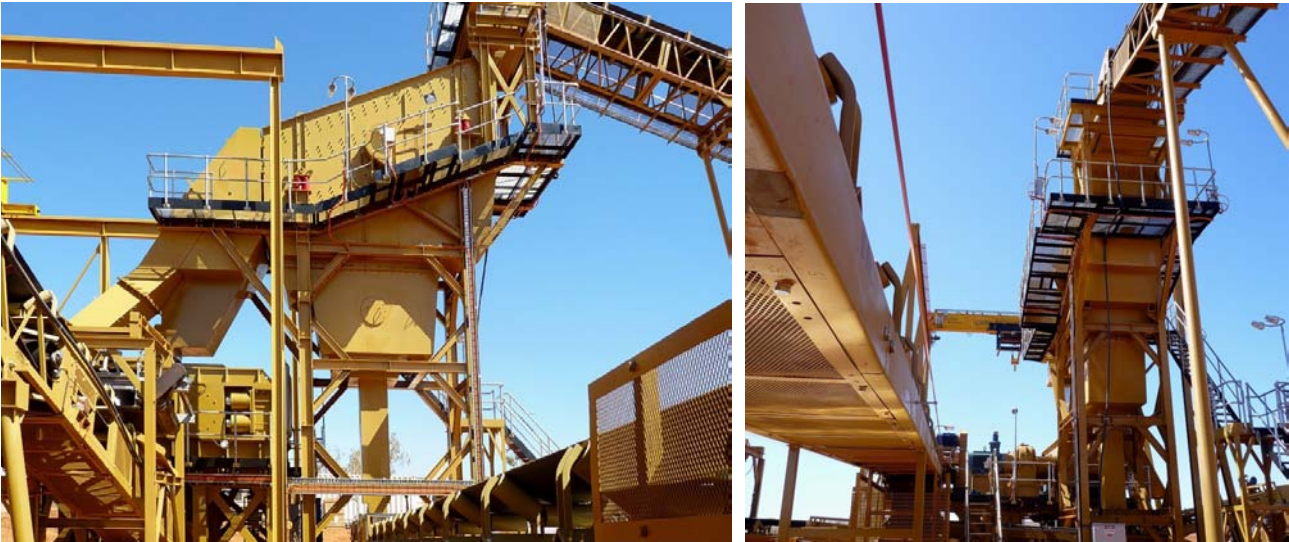
Figure 6: Crushing circuit completed and undergoing systems audit and pre-commissioning checks.
