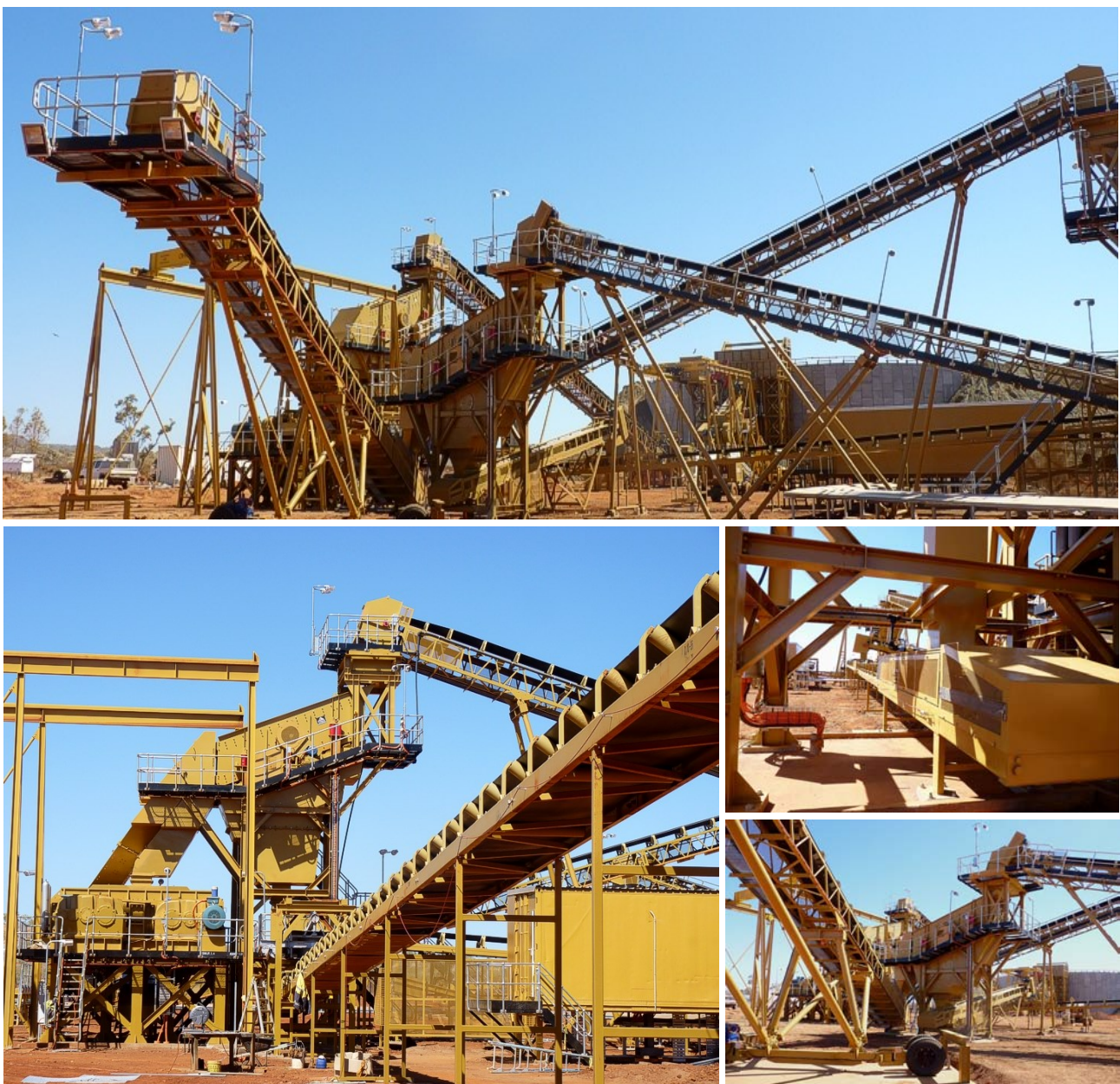
Figure 4: Crushing circuit completed and undergoing systems audit and pre-commissioning checks.
