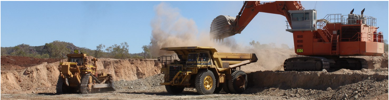
Figure 14: Mining has commenced at the RSE Pit, which will also become the PAF cell for the project once ore and waste has been removed.
