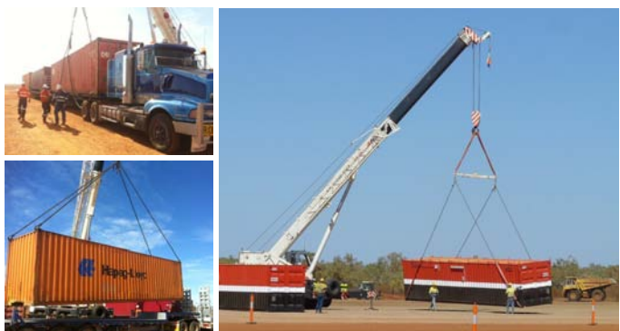
Figure 9: Heavy duty truck-crane used for various lifting needs around site.
