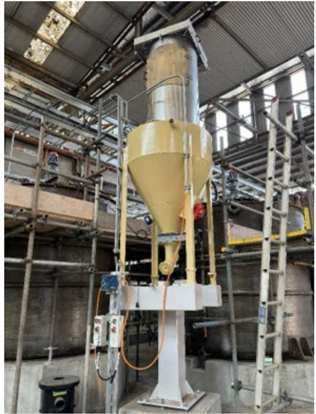
**Figure:** Hydromet piping progressing (left) Vortex pre-mixer installed and terminated (right)
