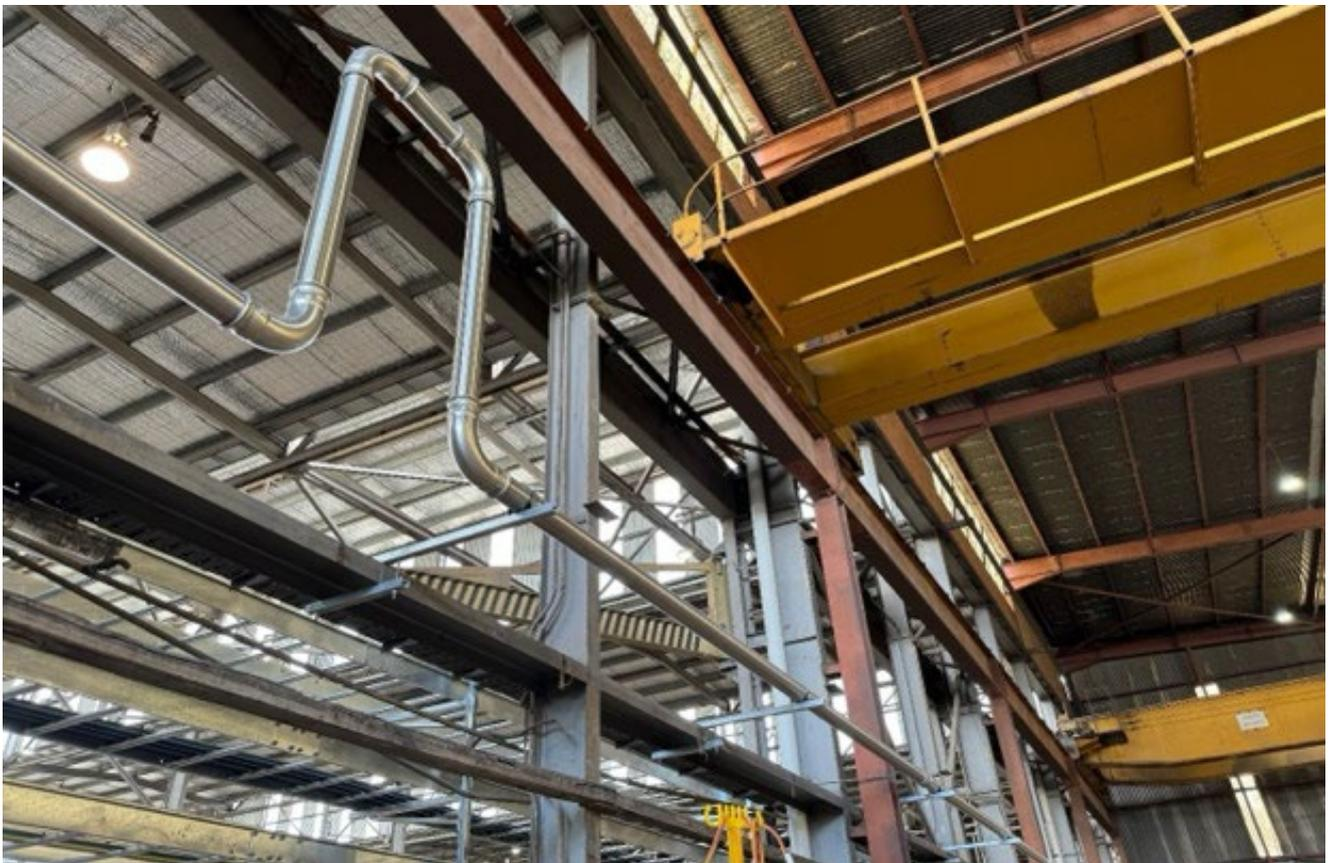
**Figure: LPG gas piping installed**
