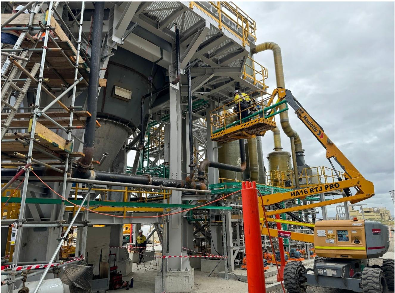
**Figure:** Spray Roaster piping installed with E&I cable installs and terminations progressing
