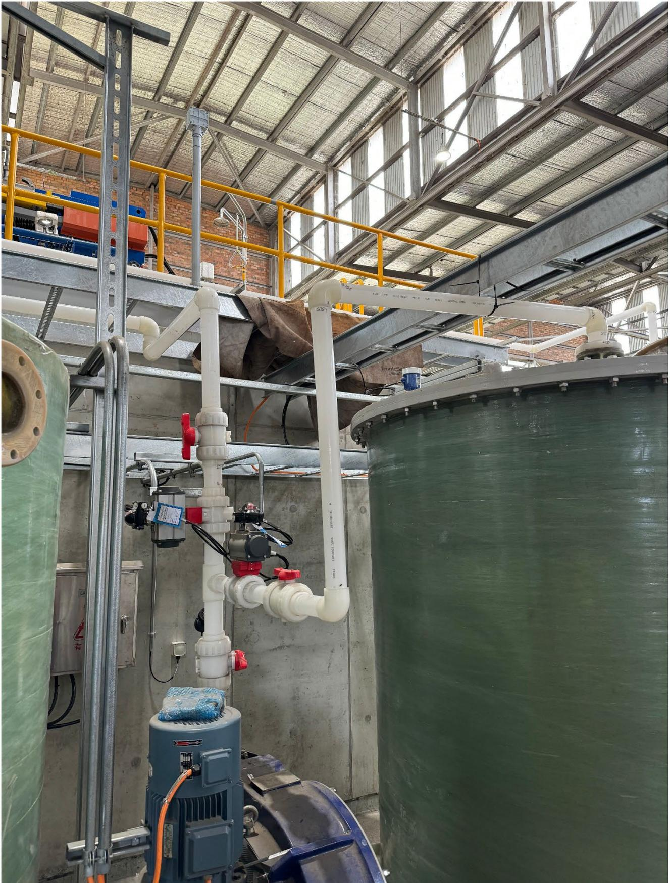
*Figure: Filter area mechanical (tanks, pumps), piping & valves and instrumentation installed*
