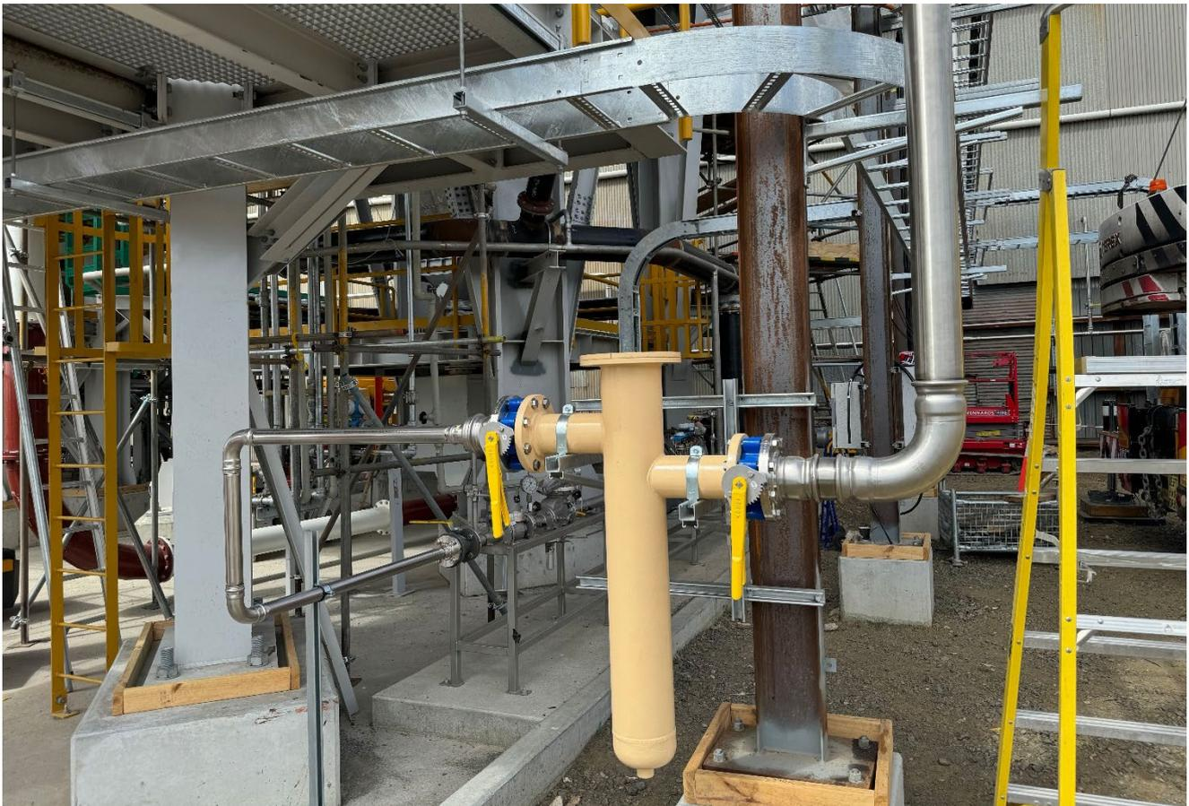
*Figure: Spray Roaster combustion fan and LPG gas piping installed*
