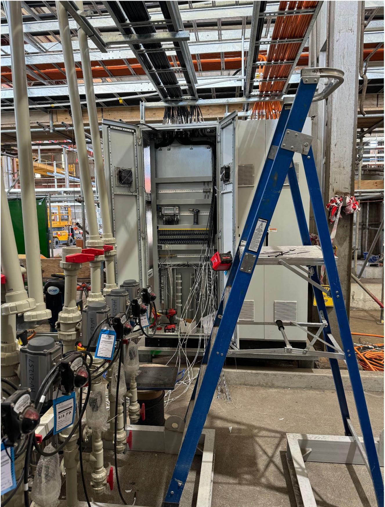
**Figure:** Terminations completed for the control cabinets in the Filtration area
