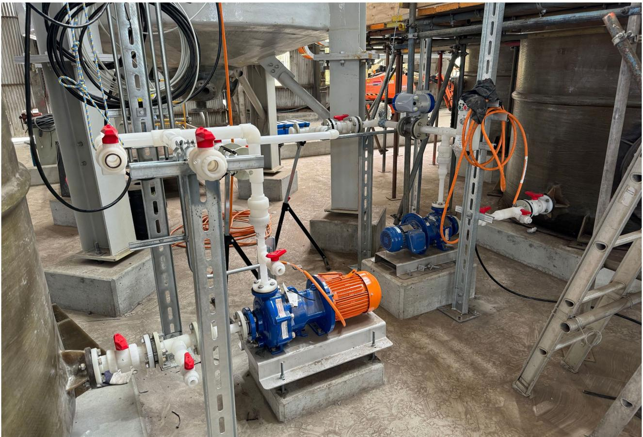
**Figure:** Thickener and PVDF tank ping installed (top) hydromet tank pump and piping installed (bottom)
