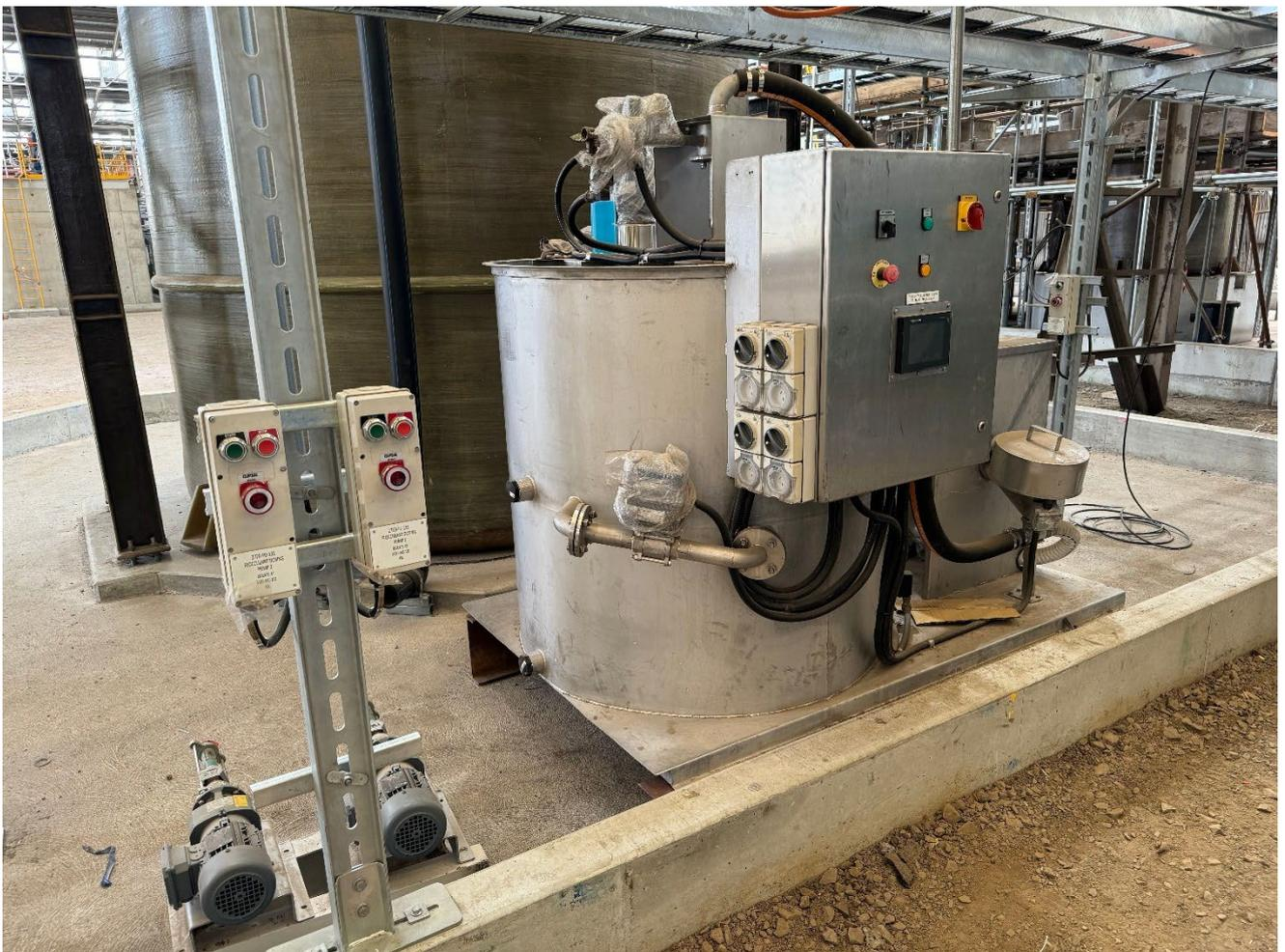
**Figure:** Air Compressor & Steam Boiler ready for commissioning (top) Flocculant package installed (bottom)
