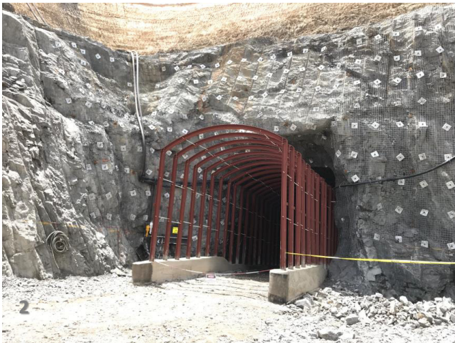
1 & 2 steel sets in the M1 South portal 3 Portal and decline operational
