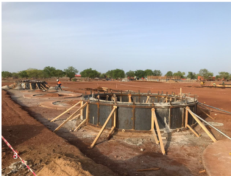
1 Generator foundations 3 HFO day tank foundations
