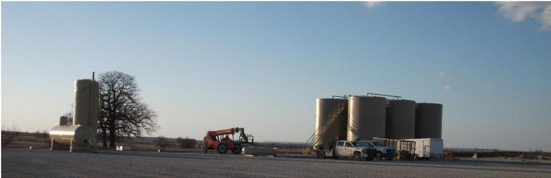
Figure 4. Rangers tank battery and separators
