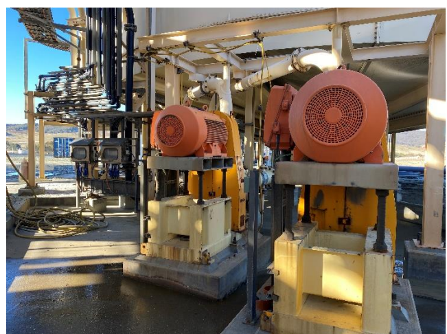
TAILINGS THICKENER PUMPS & MOTORS
