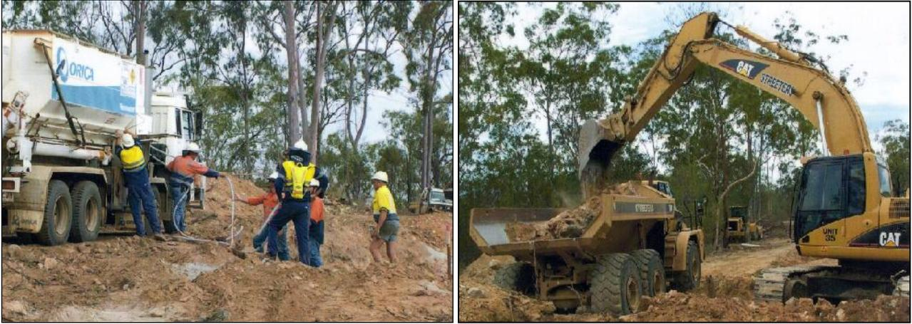
**Pictures 1 and 2:** Previous operations at Norton Gold Mine charging blast holes and mining with excavator and trucks.
