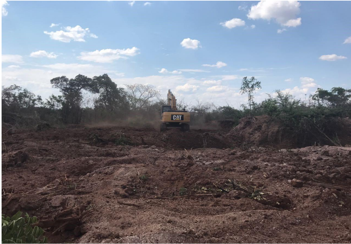
Figure 2 – Land clearing for village construction site
