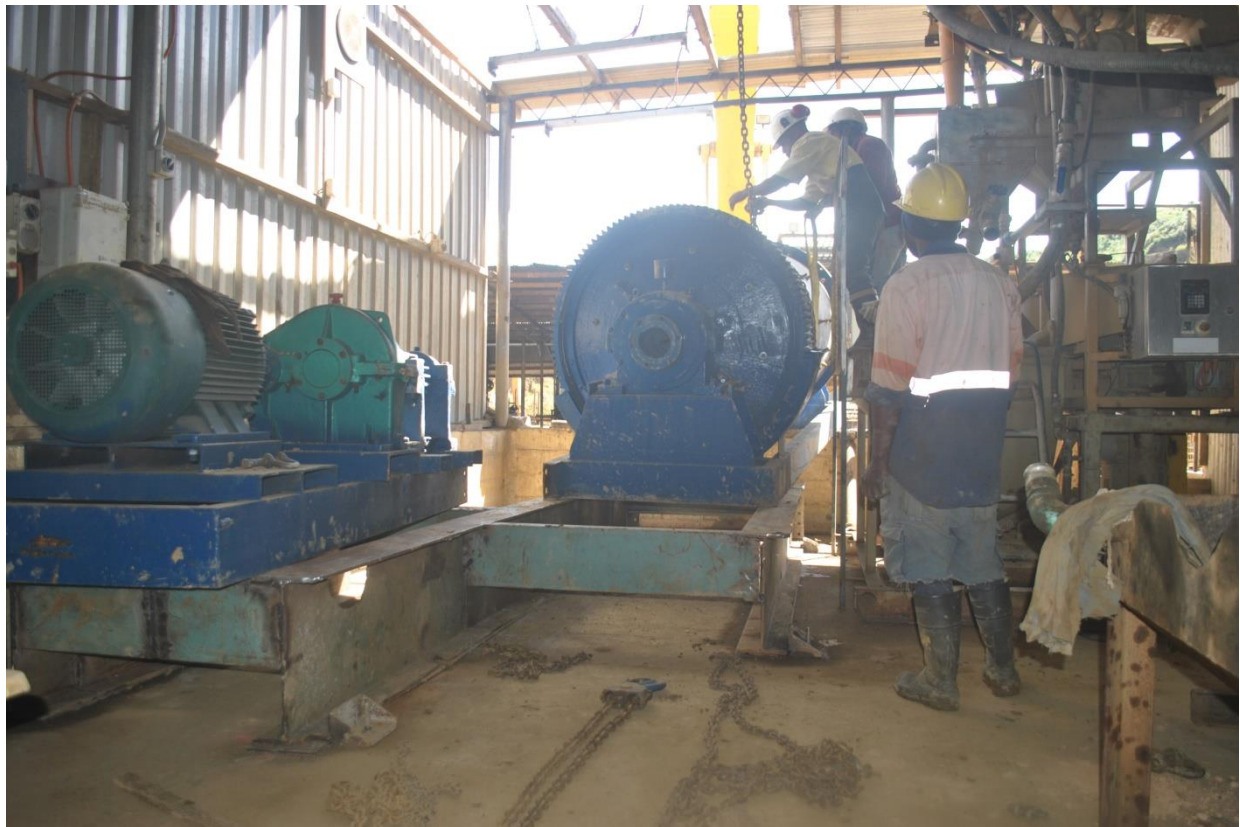
Installation of the new 5 tph ball mill
