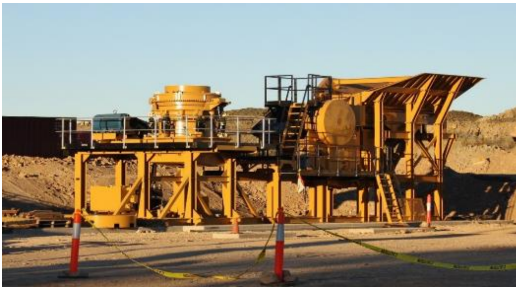
Figure 13: Primary and secondary crushers during installation in 2011.
