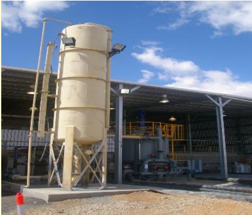
Figure 19: De-aerator and Pressure Filter in-situ at the Granite Belt Project.
