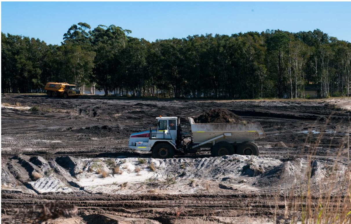
Works now underway at Latitude One, NSW Coast.
