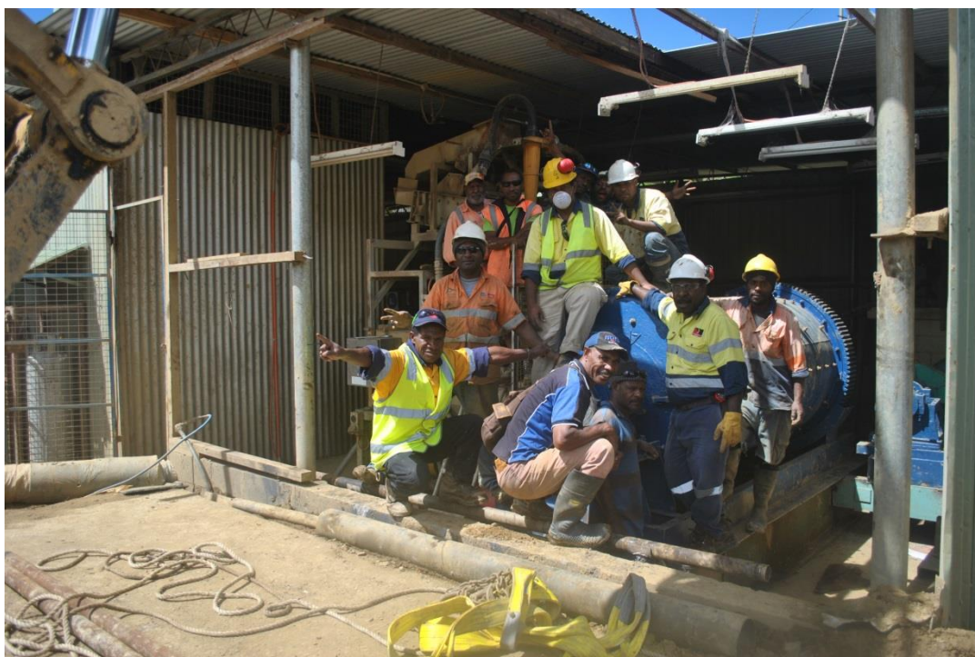
Successful installation of ball mill by the Edie Creek team
