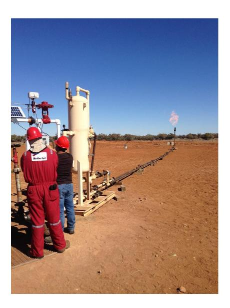
Tamarama -1 – Contractors set up surface equipment for the plunger lift system
