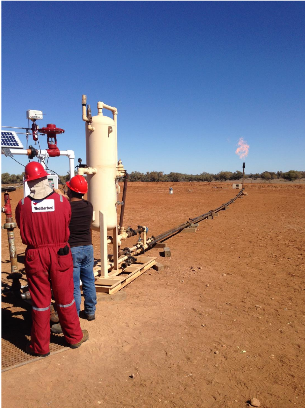
Figure 1: Tamarama -1 – Contractors set up surface equipment for the plunger lift system
