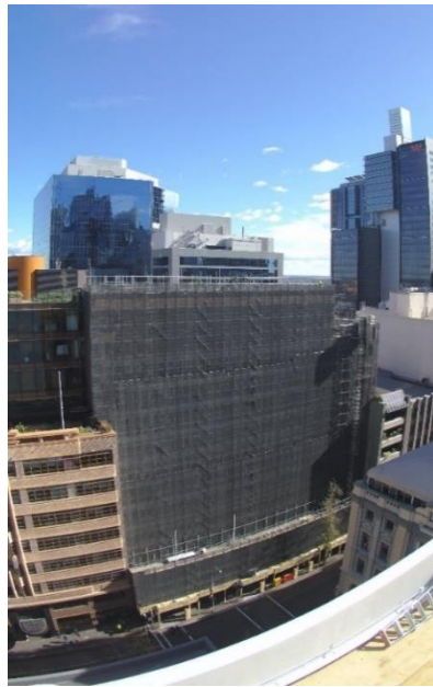
Demolition commences March 2016
