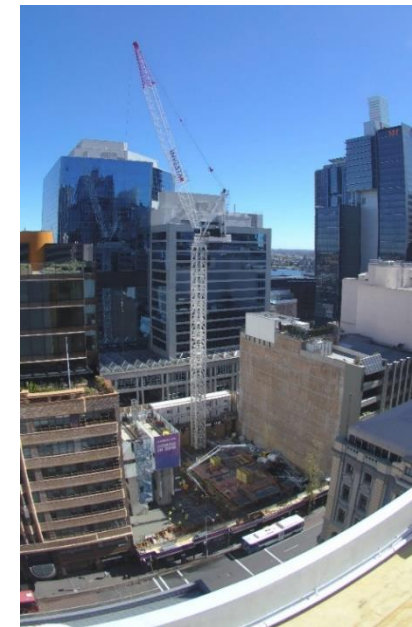
Construction underway August 2017
