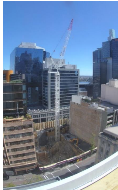
Demolition completes May 2017
