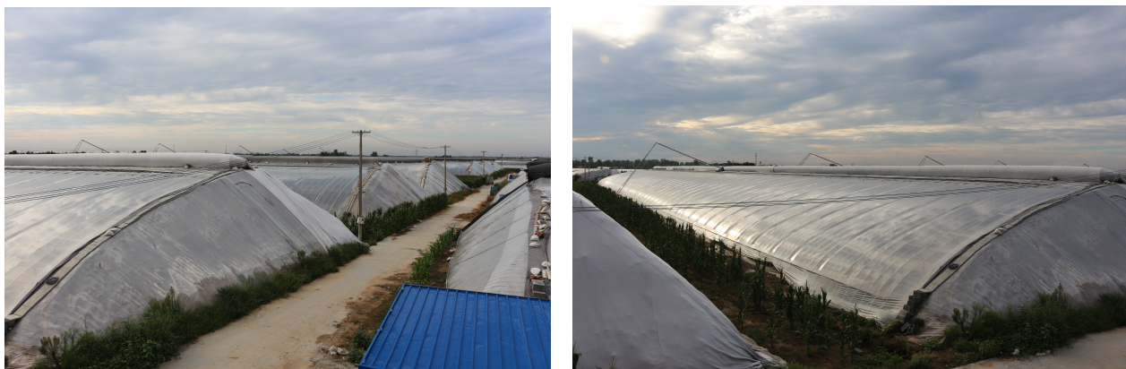
Figure 1: Newly constructed greenhouses ready for plantation from September 2017
