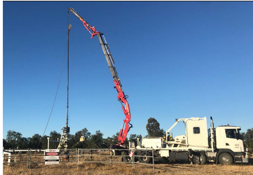
SGS performing static gradient survey on Newstead 10 well, June 2017; confirmed volume (2.3 PJ) and integrity the Newstead storage facility.
