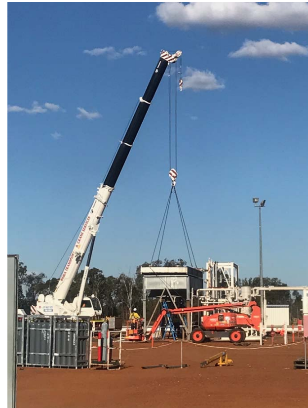
Refurbishment of Kincora Gas Plant – August 2017
