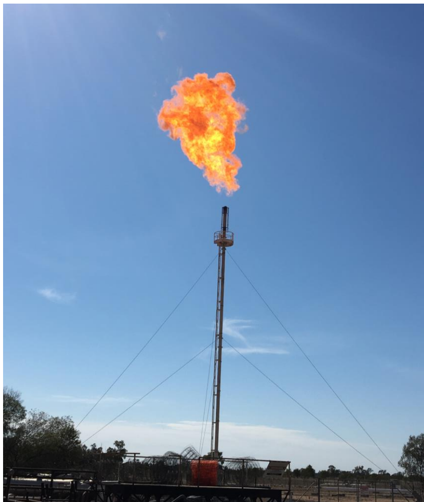
Figure 1 – Kincora Plant – flare during commissioning of dry gas circuit
