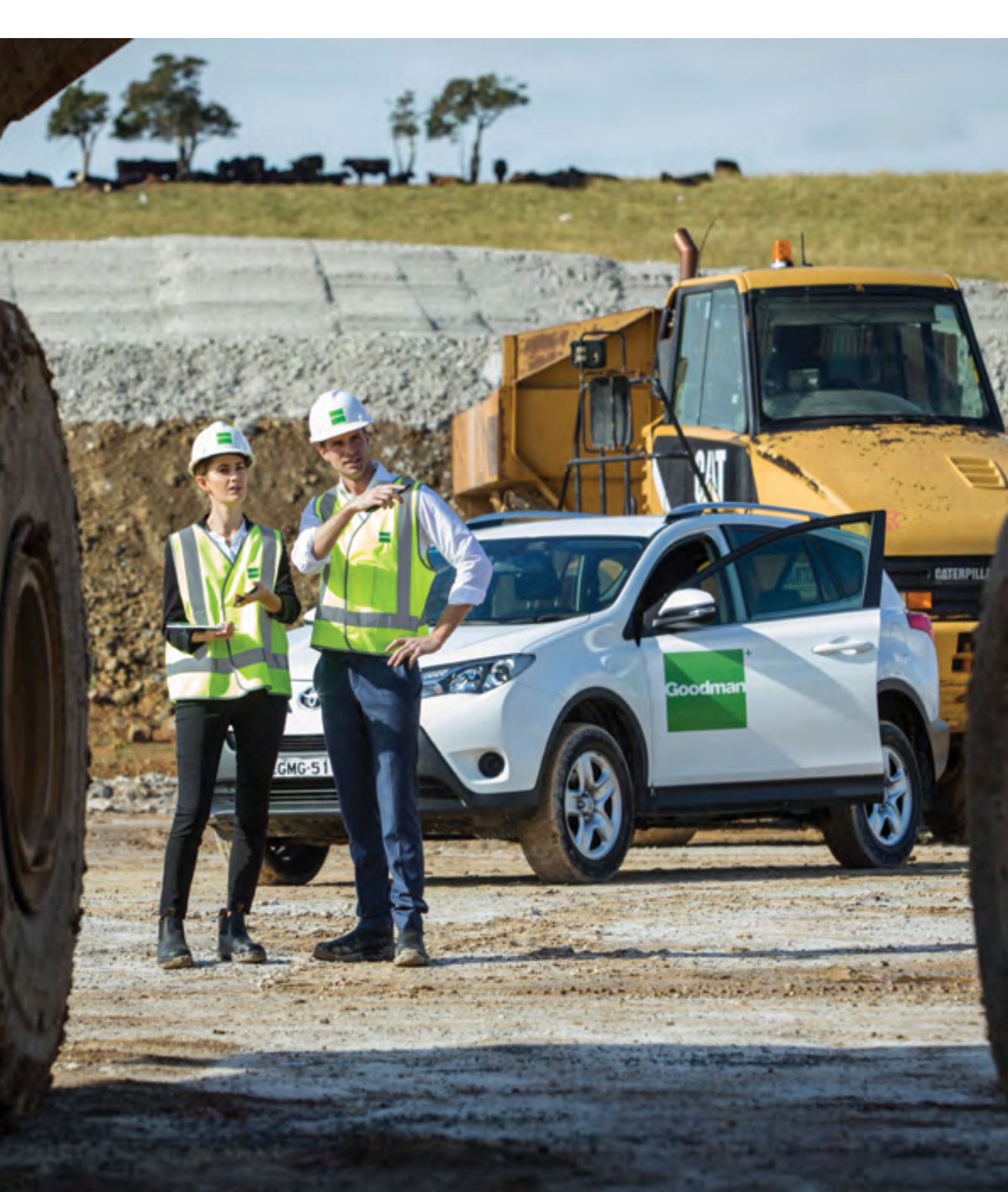
Oakdale Industrial Estate, Sydney, Australia.
