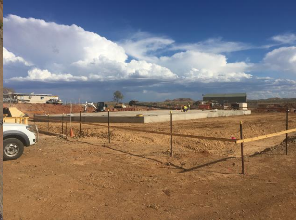
Foundations for CIL processing plant being constructed
