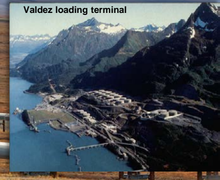
Valdez loading terminal
