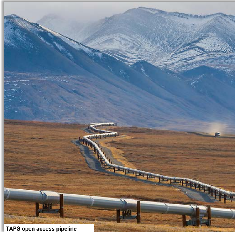
TAPS open access pipeline
