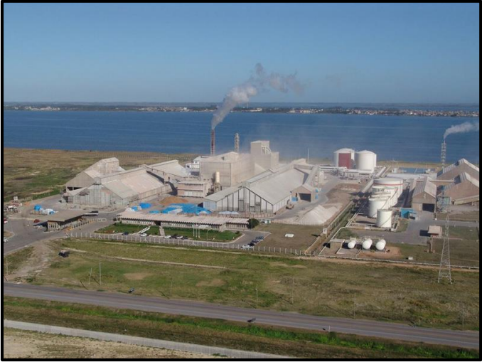
Yara's facility at port of Rio Grande
