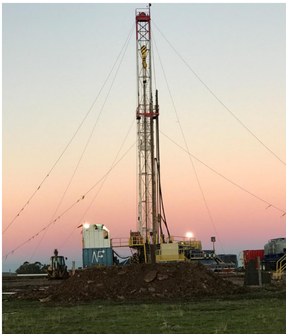
Photos - New Force rig at Cerro Padilla-1
