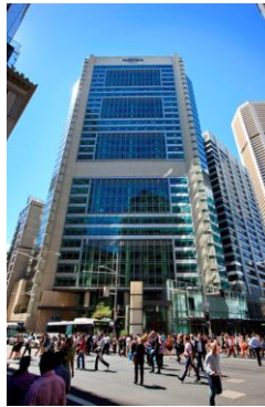
Major office refurbishment
