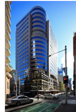
Major office refurbishment
