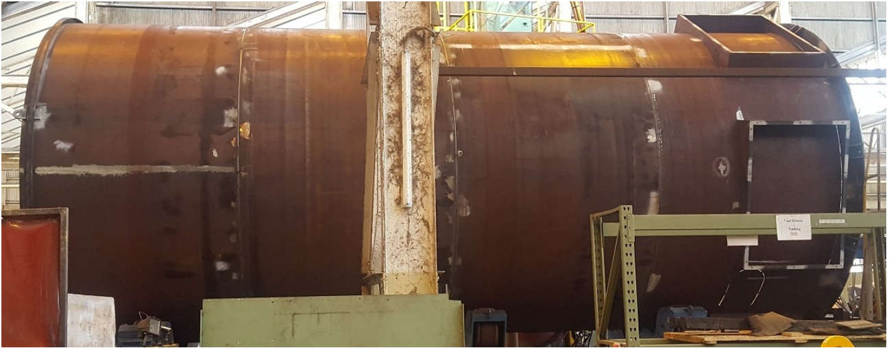
Thermal Oxidiser casing fabrication nearing completion
