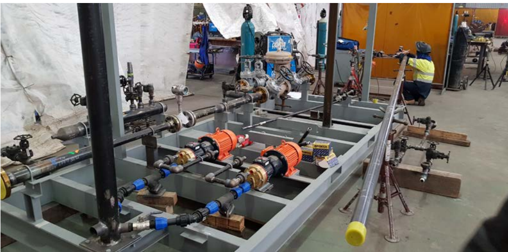
Piping and valves being installed at Ottoway Engineering
