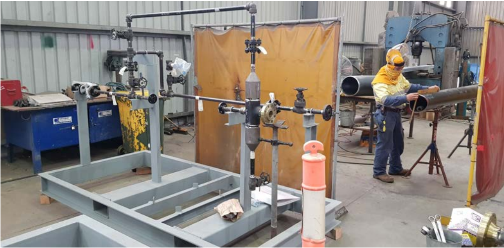
Module fabrication assembly underway
