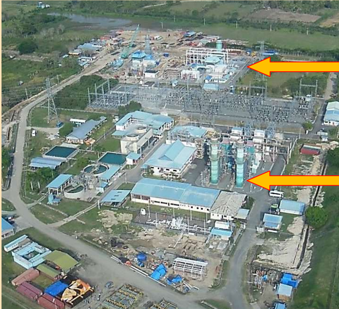
Aerial view of Sengkang Power Plant
