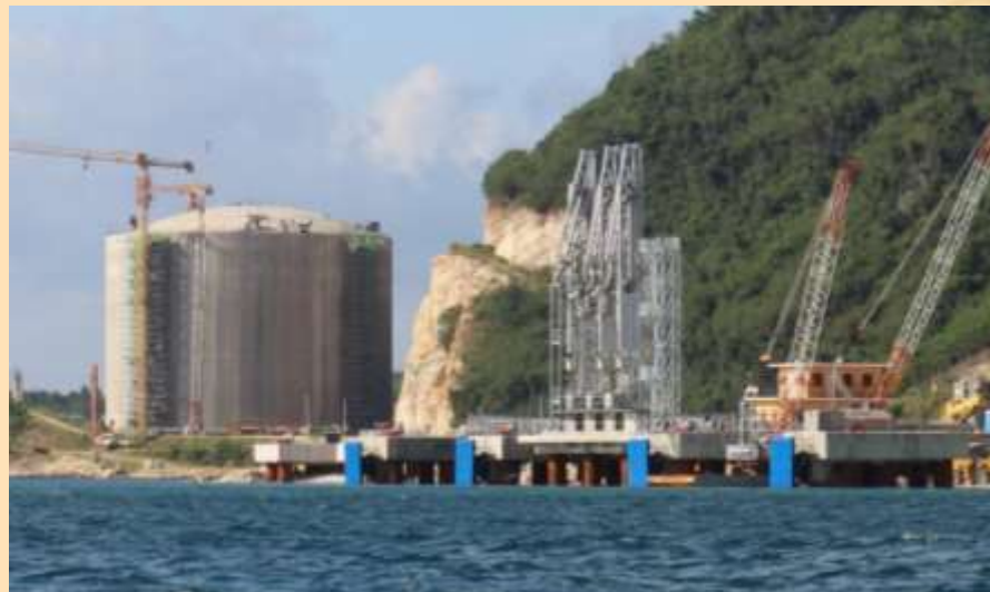
View of Jetty and Hub Terminal
