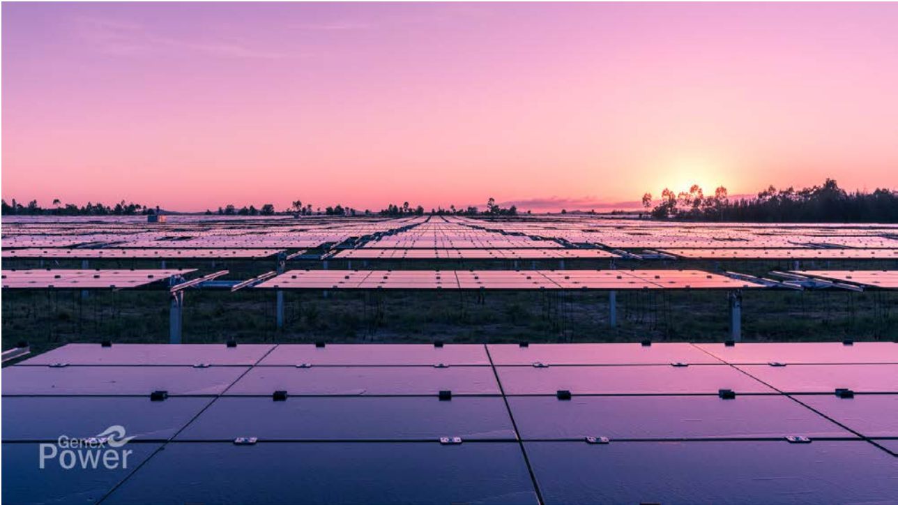
Figure 2: 50MW Kidston Solar Project (image taken October 2017)
