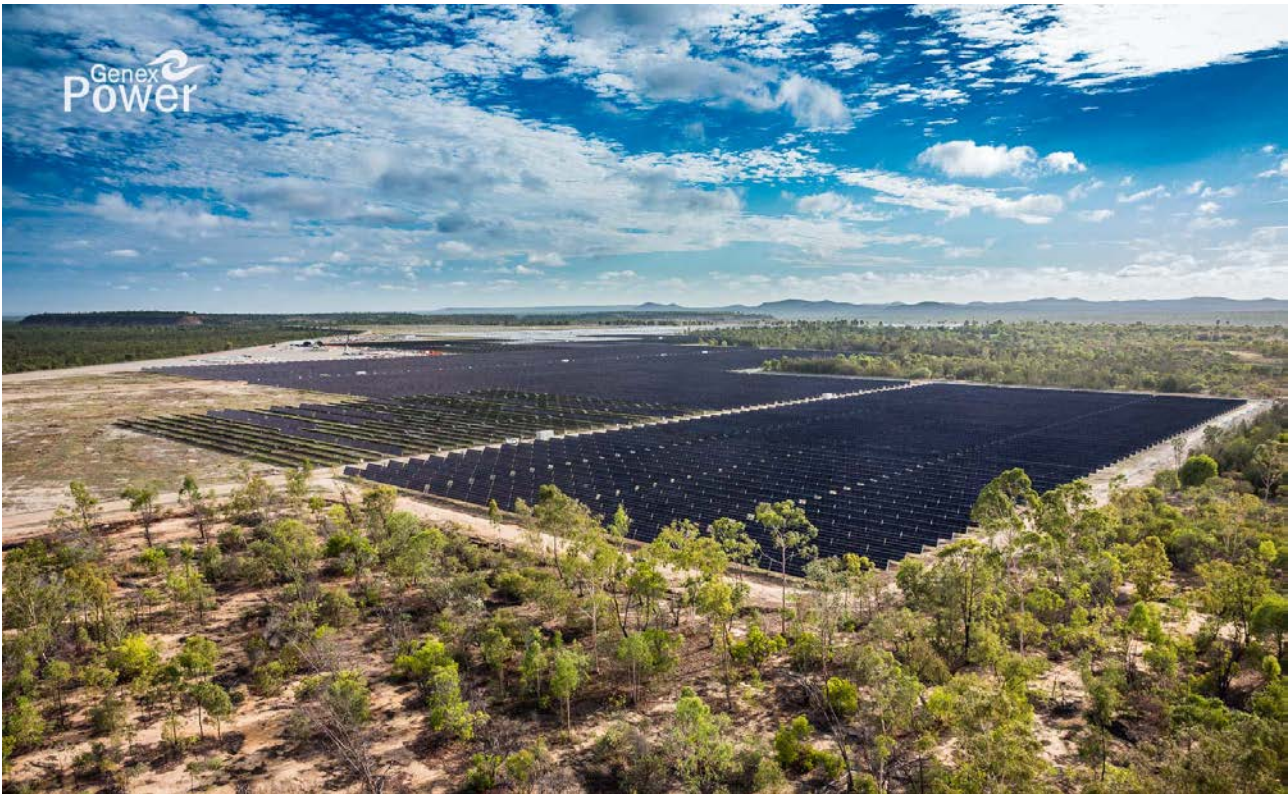
Figure 1: 50MW Kidston Solar Project (image taken October 2017)
