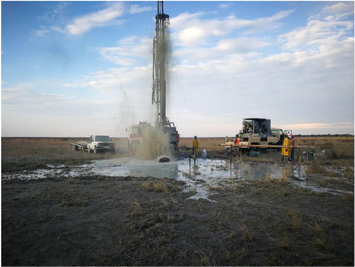
Figure 2: Drilling with strong water strikes
