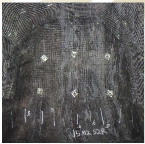
Figure 1: Challenger M2 S2 R Ore Drive face photo showing an extensive quartz package on the first ore drive on the 115m RL level.
