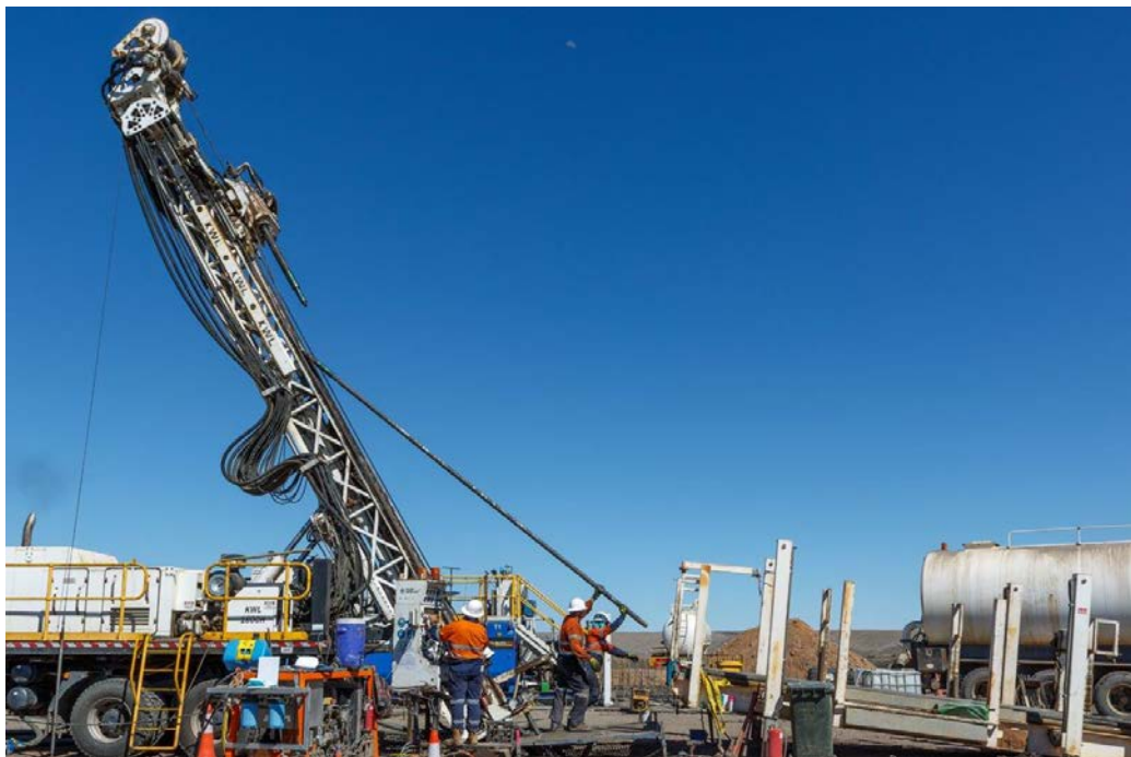
Drill rig on site at the LCEP
