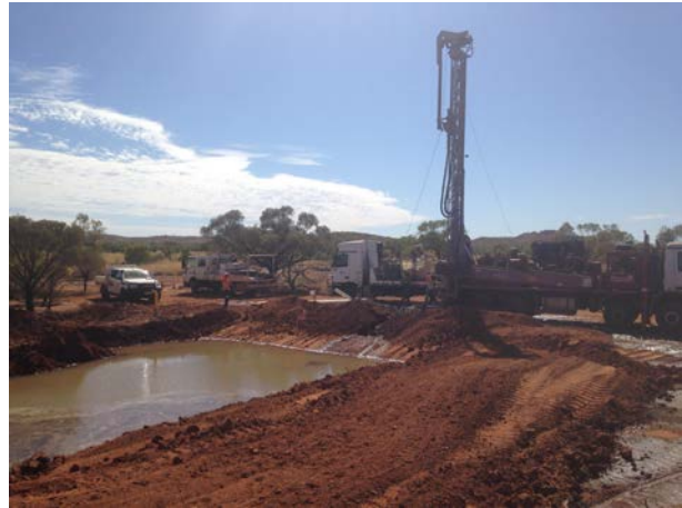
CAPTION: Water bore drilling on Ardmore Mining Lease with "turkey's nest" for pump test.
