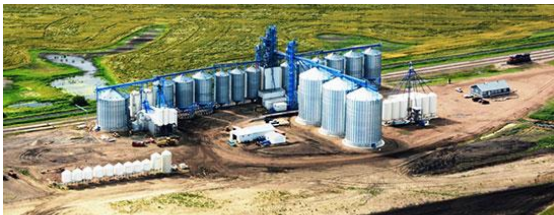
Figure 7: Providence Grain Group distribution facility
