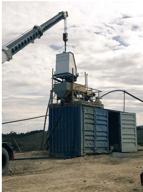
Figure 1 – DSM screen being installed prior to Jig to improve tin recovery
