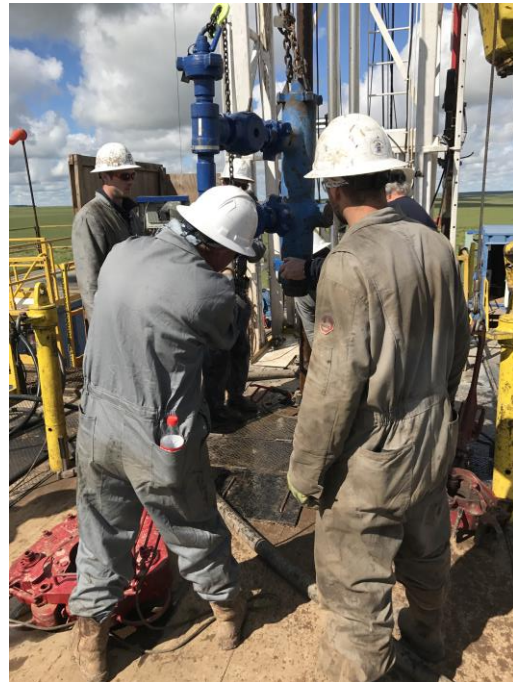
Preparations for production testing
