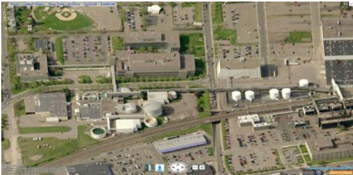
Figure 4: Huron Campus, the location of the Imperium3 New York Lithium-ion battery plant
