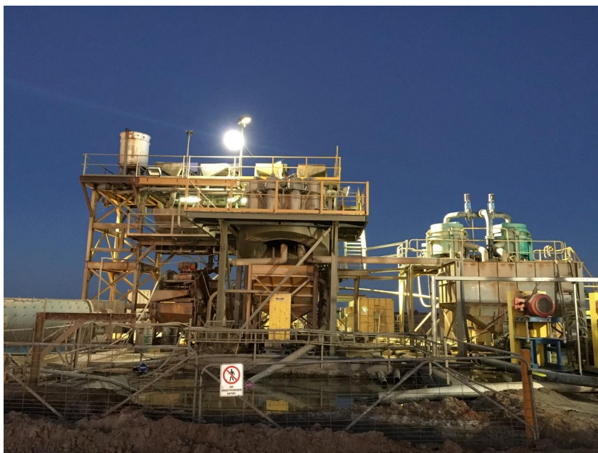
Portia Processing Plant
