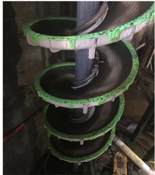
New rougher spirals targeting increased tin recovery
