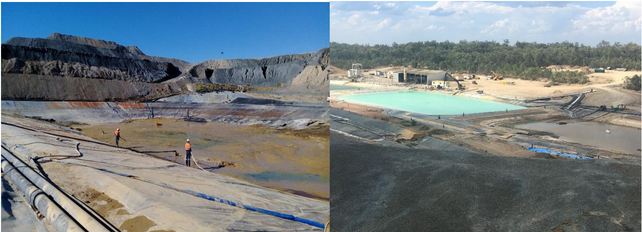
MRV Metals production crews working pregnant pond which is 80% complete, whilst our Intermediate Pond sits in circuit providing pH correction for HL 1 and 3 in preparation for the addition of Cyanide
