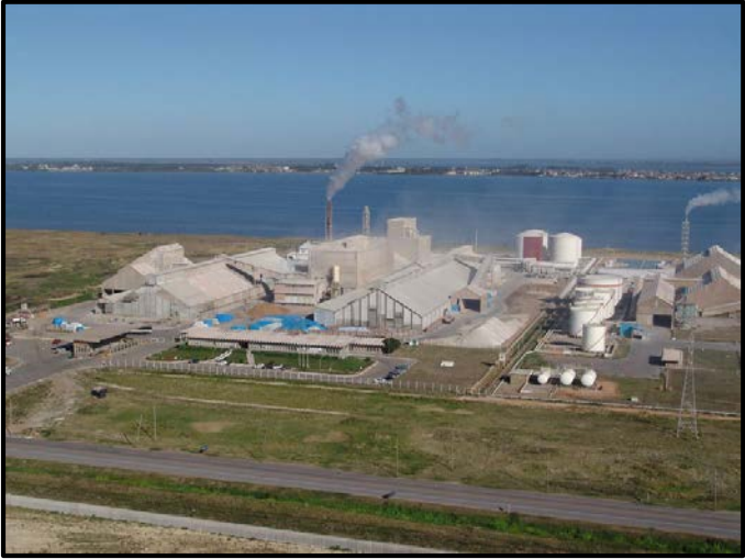
Yara's facility at port of Rio Grande
