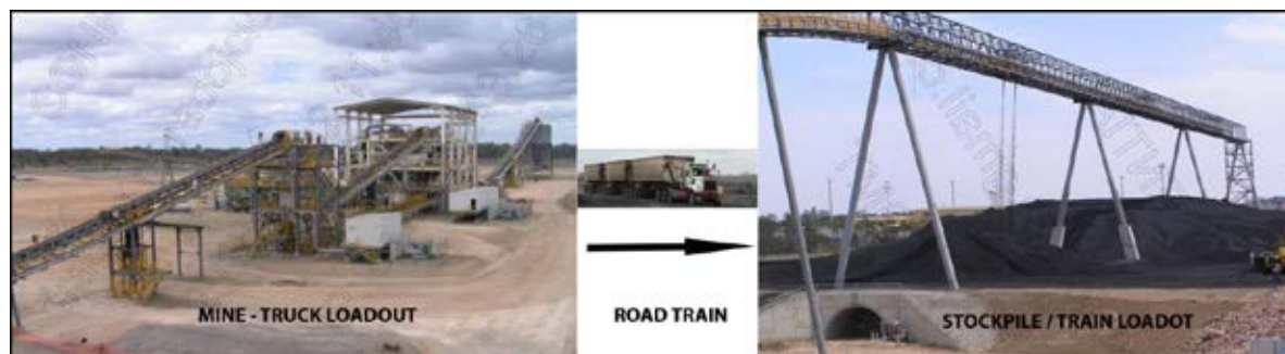
Figure 1-13: Foxleigh Mine Infrastructure Logistics
